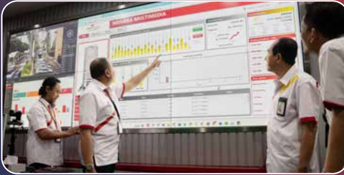
Figure 32. Building Energy Monitoring through the IBMS dashboard
