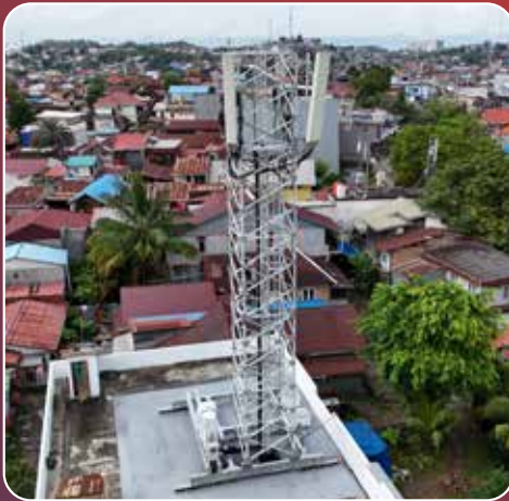
Figure 34. Glass Fiber Reinforced Polymer Tower
